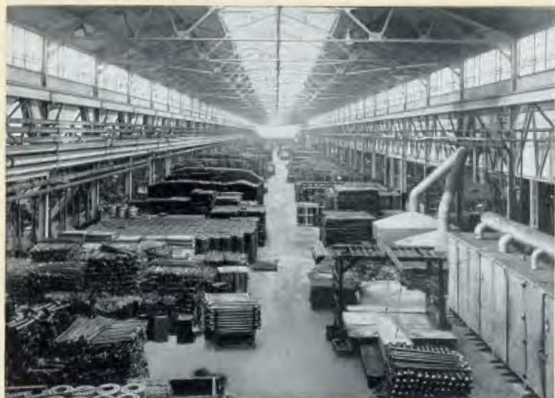
Main Factory Craneway—where rough stock is stored
